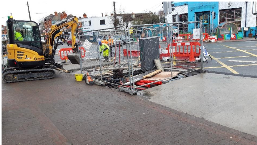
Works at Cross Guns Bridge junction
