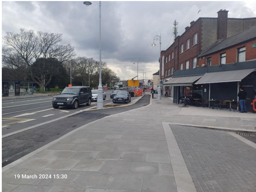
C2CC – Footway, paving and raised table pedestrian crossing at Merville Avenue
