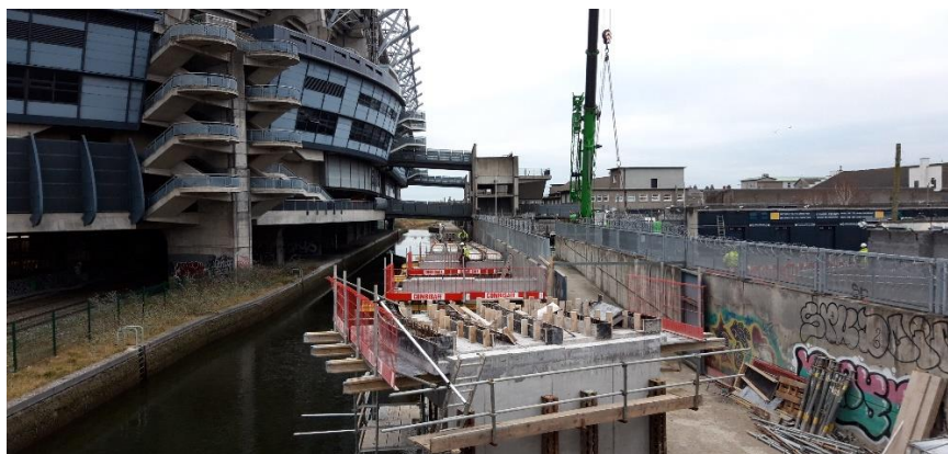
Precast ramp U- beams being lifted into place on east side of Bloody Sunday Bridge
