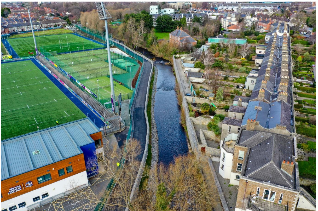
Dodder Greenway & Flood Defence Herbert Park to Donnybrook – aerial view
