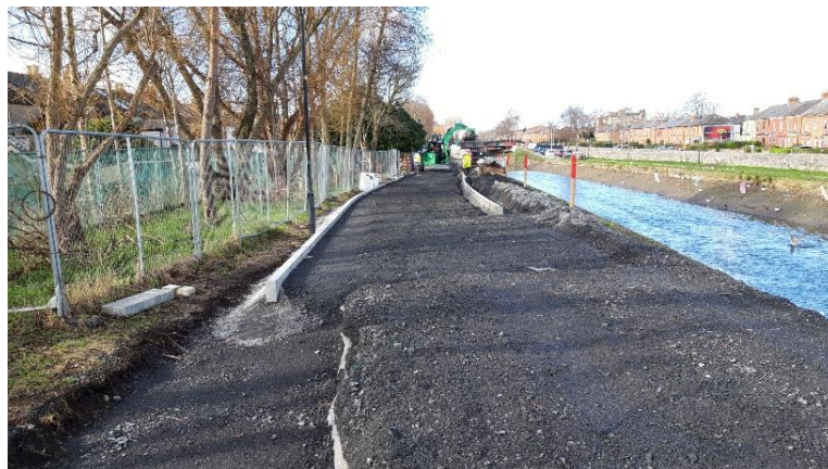
Kerbing installation on south side of canal between Binns Bridge and Lock 3
