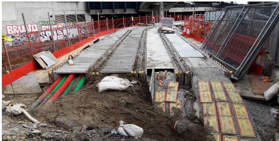
New services installed in east side ramp structure
