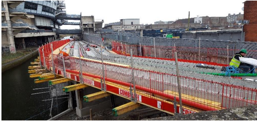
Bloody Sunday Bridge east side ramp structure
