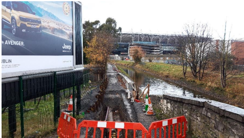
West side of Clarke's Bridge – works to resume in Q2 2024
